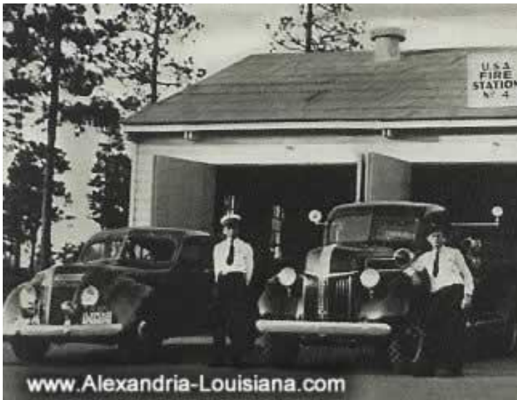
Camp Livingston Fire Station
